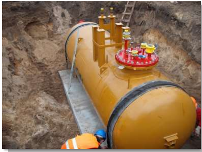
LPG filling station with underground tank - Kamien Krajski.
