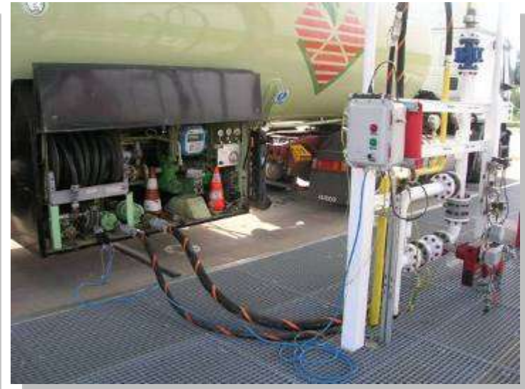
Tanktruck loading stands with automatic product loading
