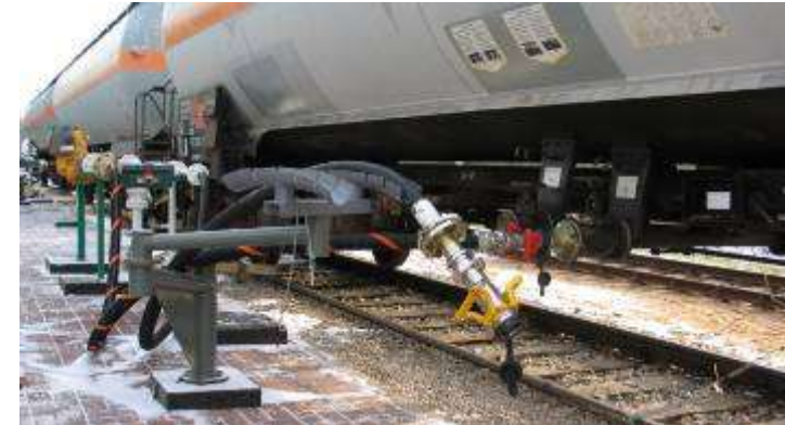
LPG railcar loading station
