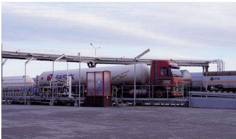
Automatic truck loading station
