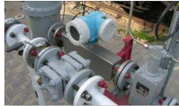
Liquid phase mass meter
