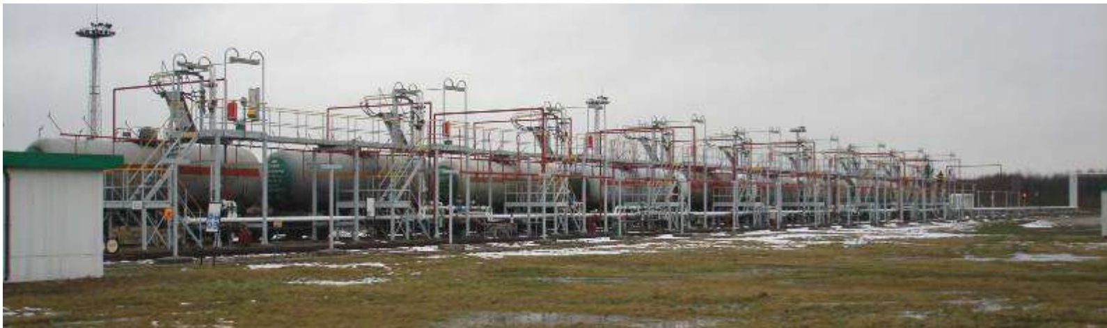
LPG railcar loading station
