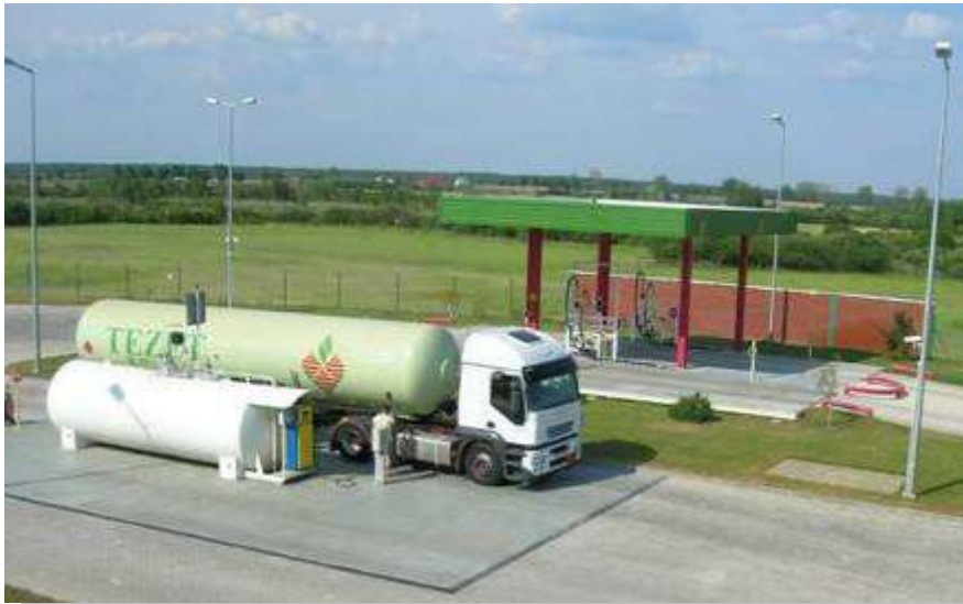
Tanktruck loading stands with automatic product loading
