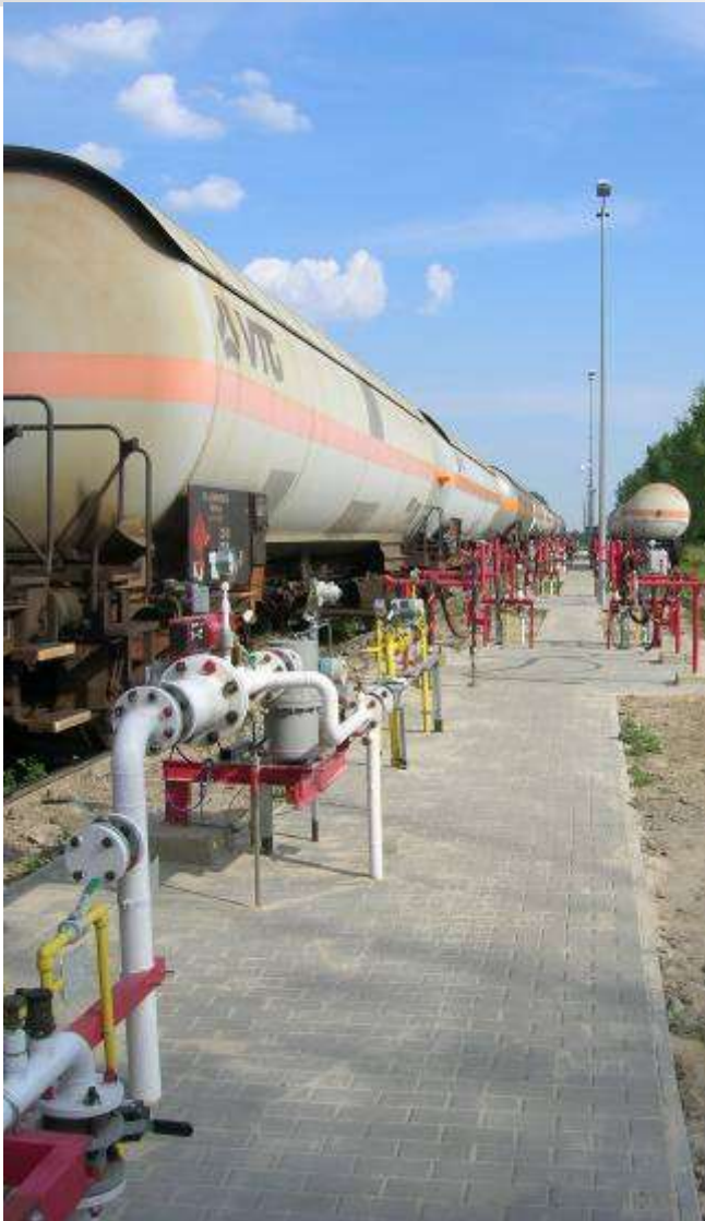
Railcar loading / unloading stands with automatic product loading
