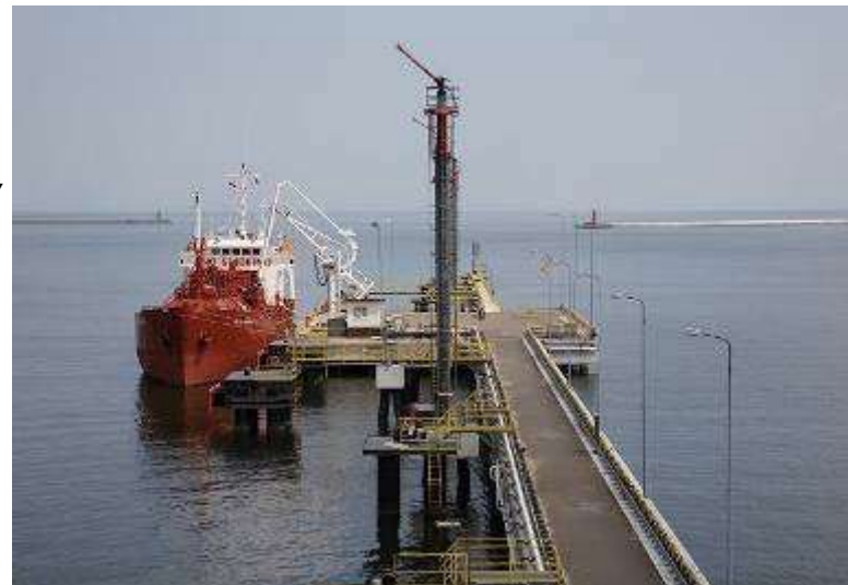
LPG sea tanker unloading station
